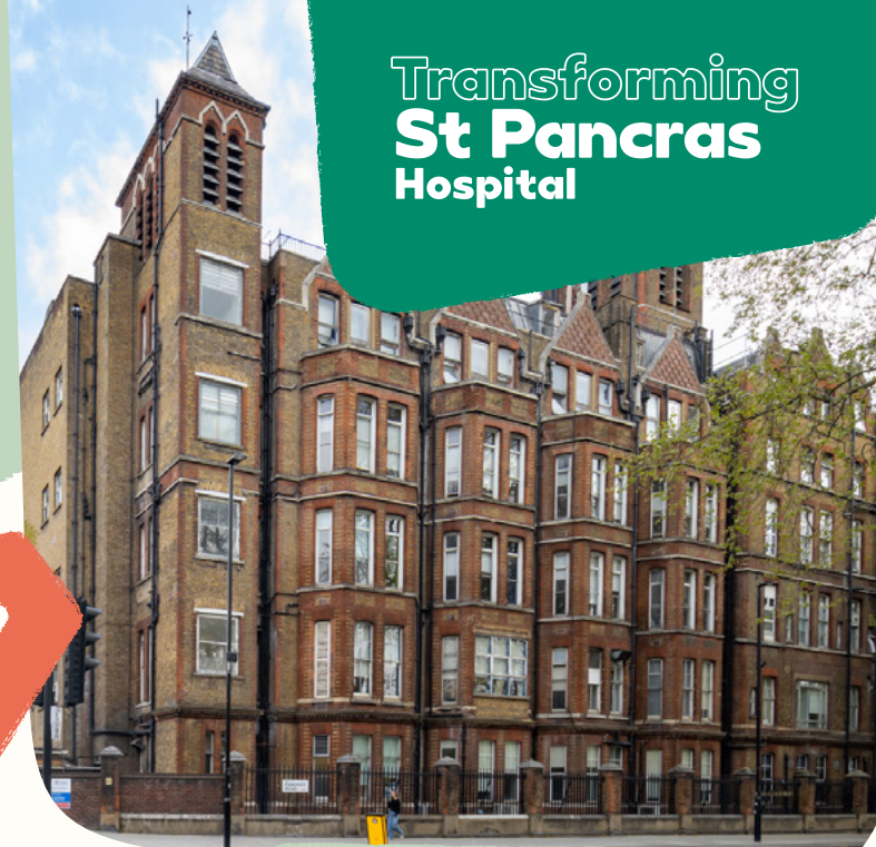
View of St Pancras Hospital from Pancras Road
