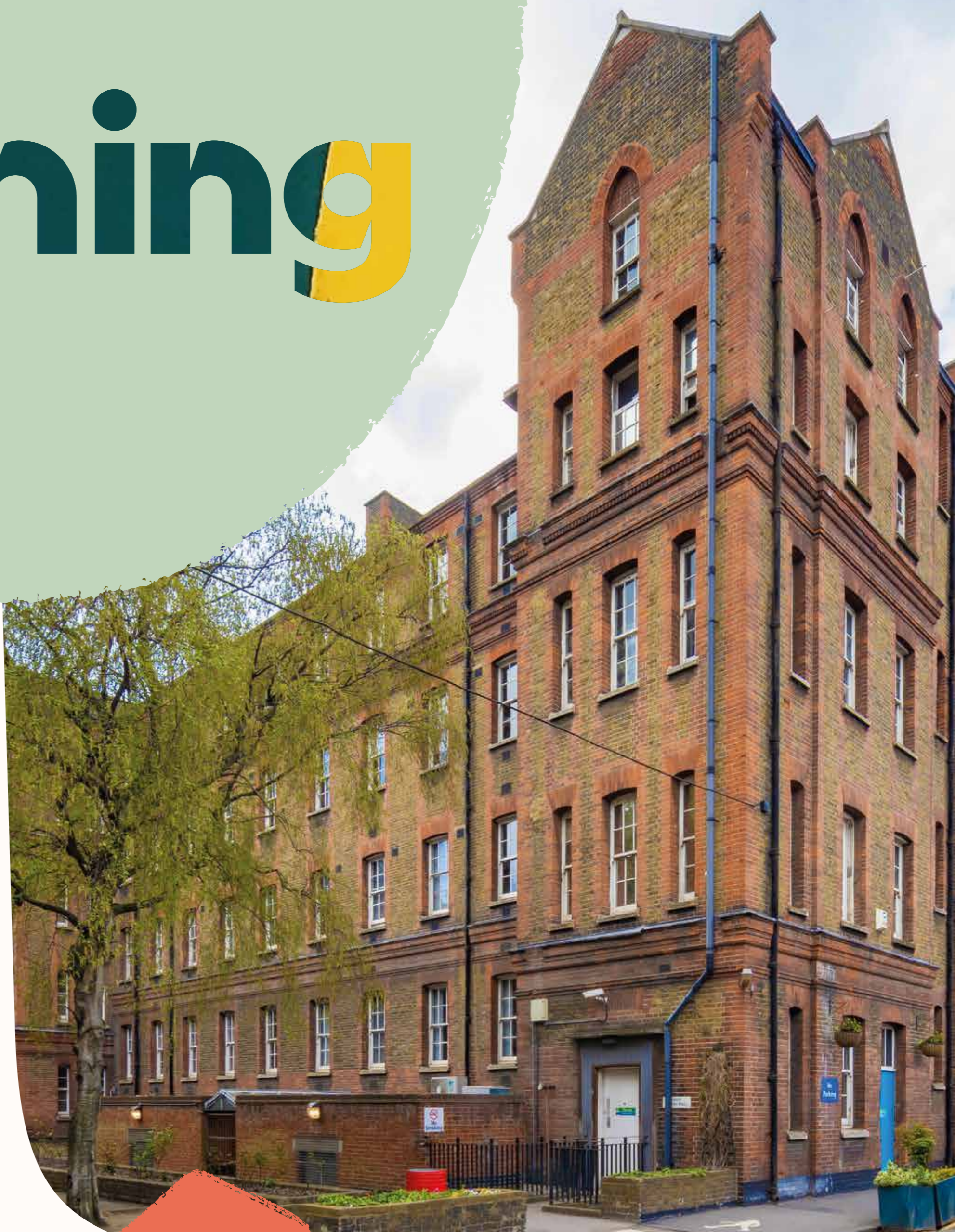
An existing building on the St Pancras Hospital site
